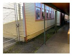
**Note:** Moss was noted on the pavement and discoloration to the lower wood skirting at the northeast corner. This indicated increased moisture in this area. It is recommended that these areas be cleaned and appropriately sealed to minimize facility damage.
