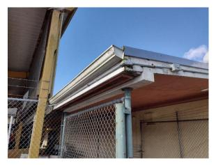
Note: Moss was noted in the corners and around the gutters. It is recommended that these areas be cleaned and appropriately sealed to minimize facility damage.
