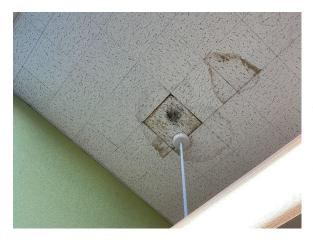
Note: Areas of discoloration were noted on the ceiling tiles from previous roof leaks. There is no evidence of any growth and no moisture detected at the time of inspection. This being the most discolored, it was removed to inspect underneath. No growth and only minor discoloration was noted behind the tile.
