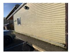
**Note:** Grass and moss had grown in the cracks of the walkways and between the walkway and foundation. Moss was also noted growing on the metal flashing at the base of the lap siding. It is recommended that these areas be cleaned and appropriately sealed to minimize facility damage.
