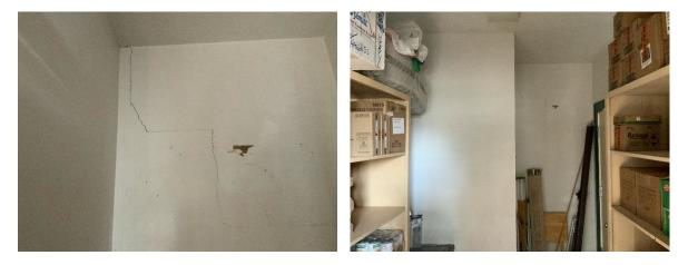
Note: There is a crack in the plaster wall of the storage room adjoining the pantry storage room. It is recommended the crack be filled and sealed to minimize any progressing damage.
