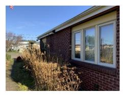
**Note:** Observed the vegetation around the building is within 1 foot from the exterior walls. It is recommended that the landscaping be trimmed back to provide 2 feet of clear space.
