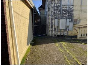
Note: Grass and moss had grown in the cracks of the walkways and between the walkway and foundation. It is recommended that these areas be cleaned and appropriately sealed to minimize facility damage.
