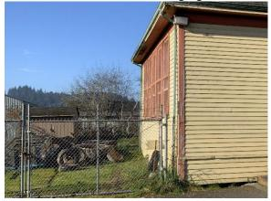
Note: Moss And discoloration was noted on the soffits, facia, and around the gutters. It is recommended that these areas be cleaned and appropriately sealed to minimize facility damage.
