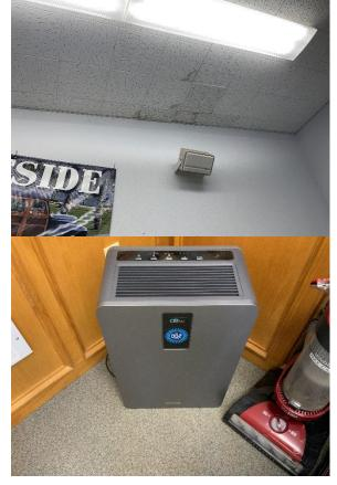
Note: Areas of discoloration were noted on the ceiling tiles from previous roof leaks. There is no evidence of any growth and no moisture detected at the time of inspection.
