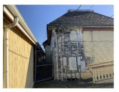
**Note:** Paint deterioration has been noted on the northwestern corner of the building. Based on the age of the building the exterior should be assessed or assumed to contain lead-based paint. ACS recommends a lead-based paint certified contractor be contacted to assess the damaged areas and encapsulate, remove or repair as required.
